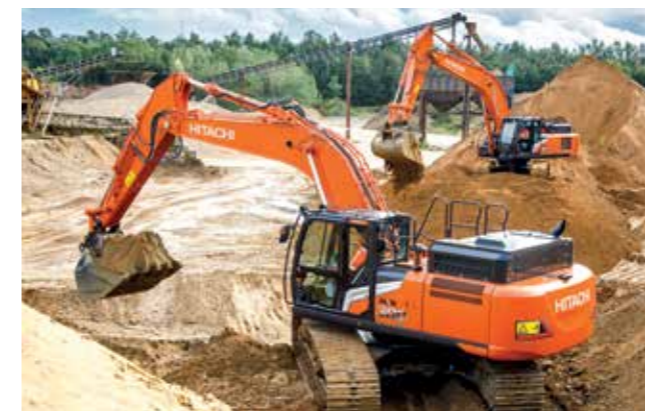
Zaxis medium excavators
